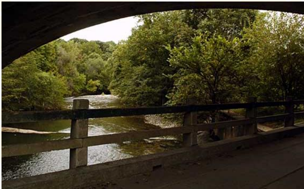
A VIEW FROM UNDER THE HARFORD ROAD BRIDGE
