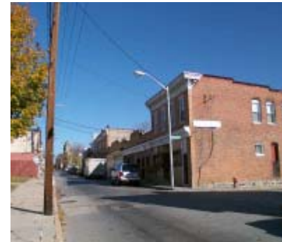
Dilapidated commercial properties on the 4000 block of Old York Road
