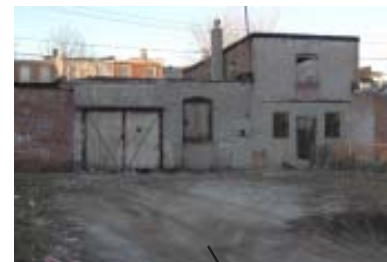
Condemned house at 628 Dumbarton (far left), dumping (lower left) and dilapidated garages (immediate left) adjacent to each other along Dumbarton and alley
