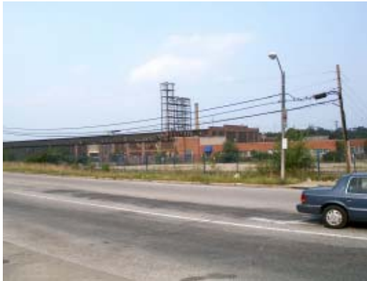
The former Anchor Fence property at Eastern Ave. and Kane Street has been approved to be redeveloped as a full service grocery store with additional commercial spaces.
