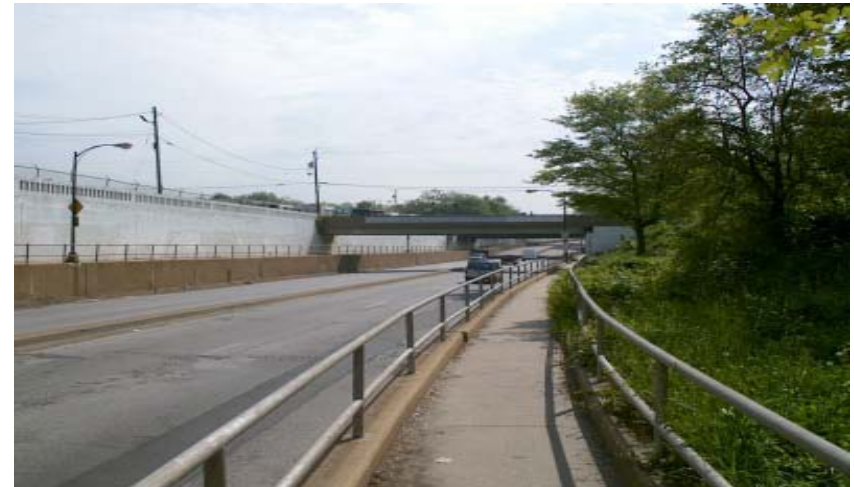
Existing condition of Eastern Avenue gateway into Greektown
