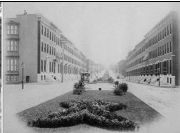
Figure 10: Olmsted-designed Fulton Avenue median
